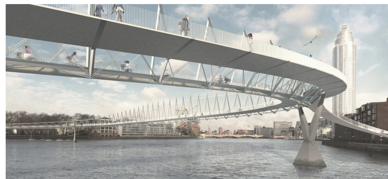
View from the southern bank looking downstream
