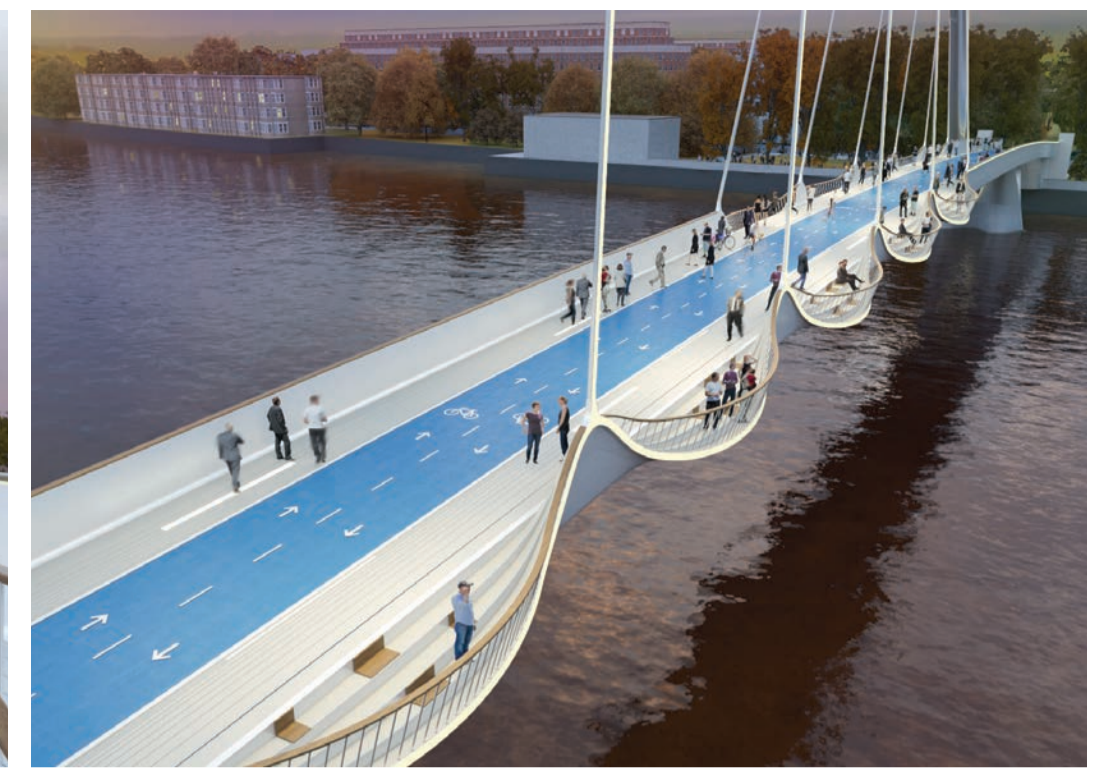
Deck and tension cables + viewing balconies
