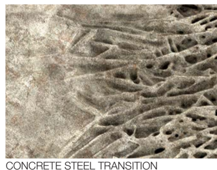
CONCRETE STEEL TRANSITION
